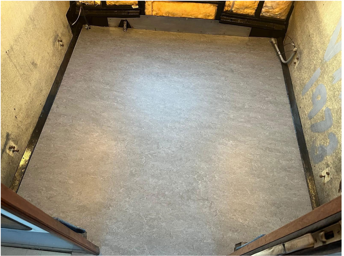
New linoleum laid in one of the compartments
