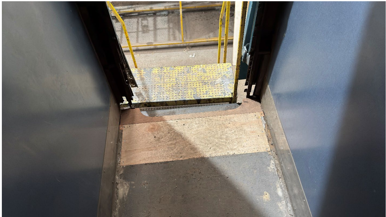
Pictures showing repairs to the floors, including new hardwood door step inserts
