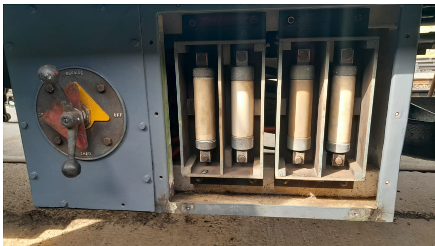
Finished supply case after welding repairs to damage front completed
