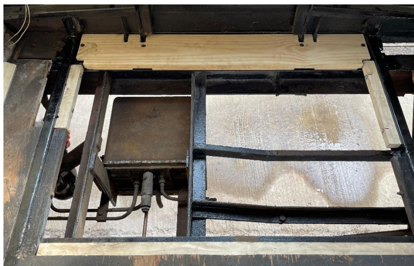
Compartment floor bearers being replaced
