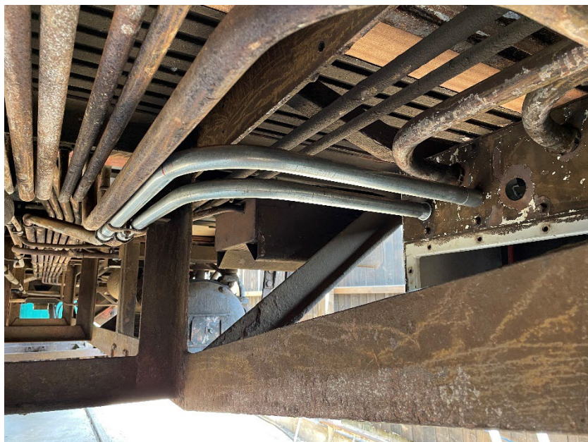
New conduit fitted to replace sections damaged when cable was stolen (above and below)
